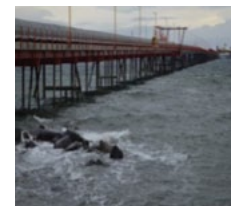
Coal-loading pier, Otway Channel
